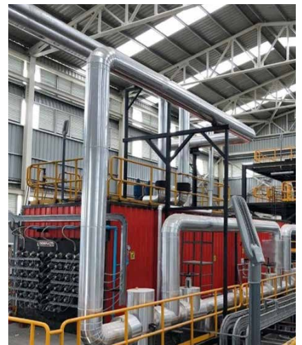
Thermax's reciprocating grate Combipac® boiler
