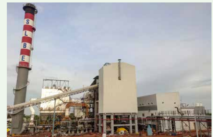
The 5.3 MW cogeneration plant for a leading ethanol manufacturer in Tamil Nadu
