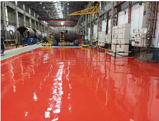
The new floor after the installation of polyurethane (PU) concrete flooring
