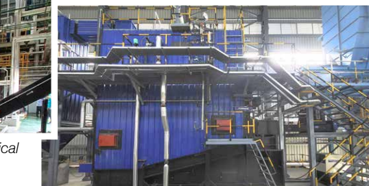
The 6 TPH UltraPac boiler for a leading food processing facility
