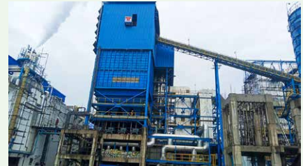
An 8 MW cogeneration plant for a grain-based ethanol manufacturer in West Bengal
