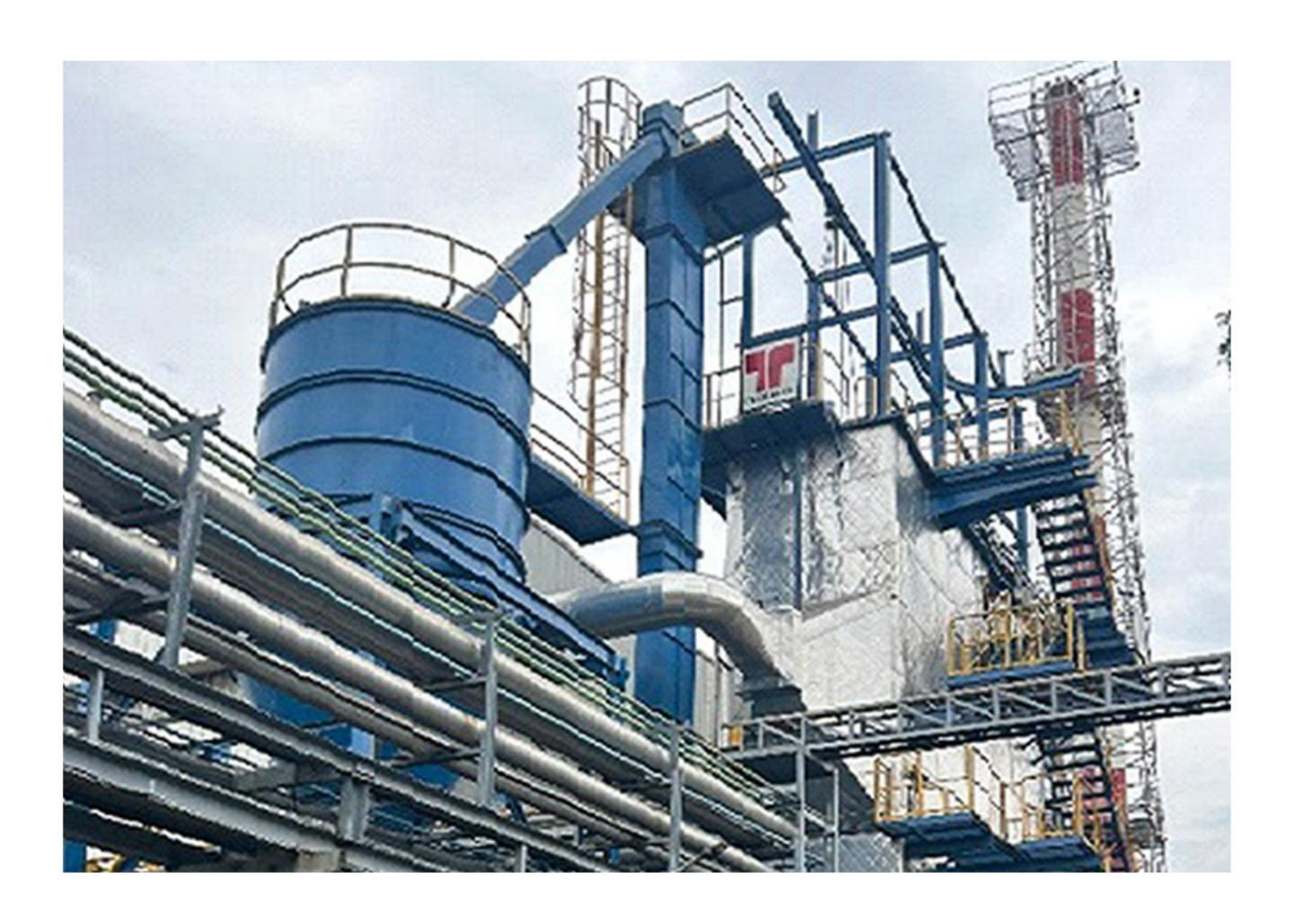
Thermax delivered an end-to-end turnkey solution centered on a 10 TPH UltraPac biomass boiler, featuring advanced Reciprocating Grate Technology. The solution incorporated:
