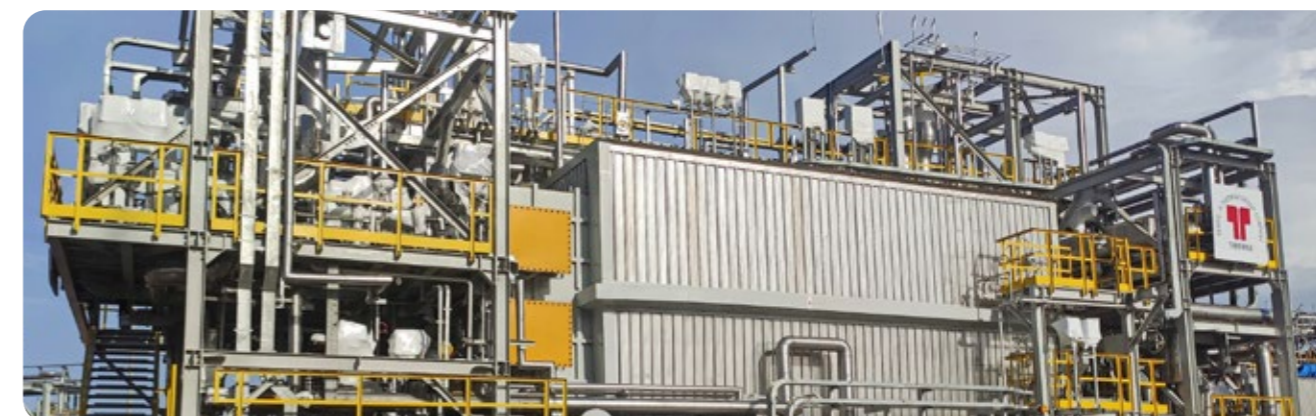
■ 3x80 TPH modularised plug-and-play boilers supplied to a major refinery in Iraq
