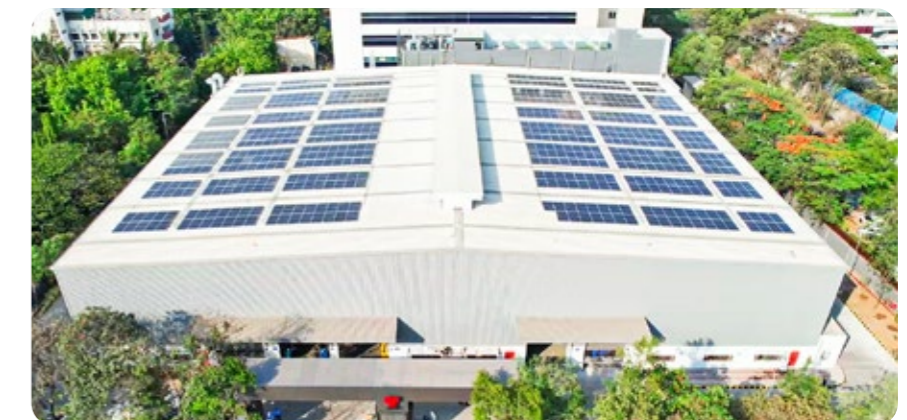
Aerial view of the new water and wastewater solutions manufacturing unit
