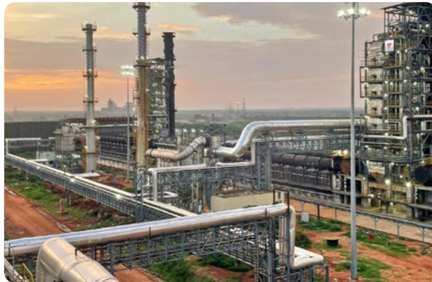
The 20 MW captive power plant commissioned for a leading alloy steel manufacturer in South India
