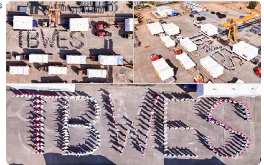
TBWES successfully shipped out its first consignment consisting of a fleet of 17 assembled modules for a leading waste to energy technology OEM in Europe
