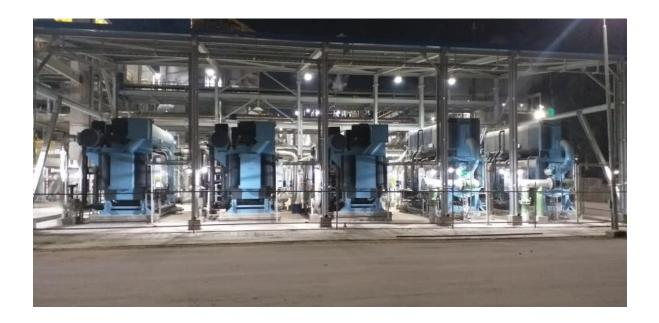
Thermax's smart and innovative solution for inlet air cooling application provided for CFCL improves the turbine and PAC capacity. As a result, the capacity is maintained throughout the
