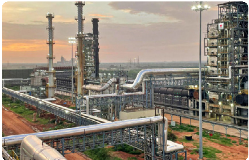
The 20 MW captive power plant commissioned for a leading alloy steel manufacturer in South India
